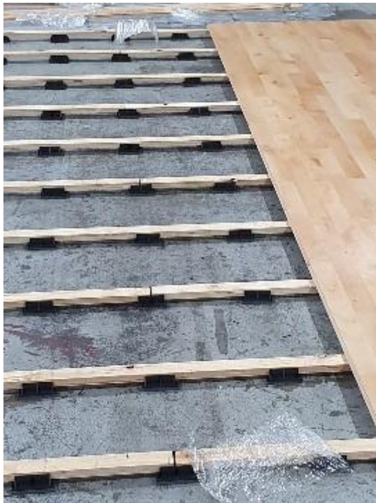
Floor being built
